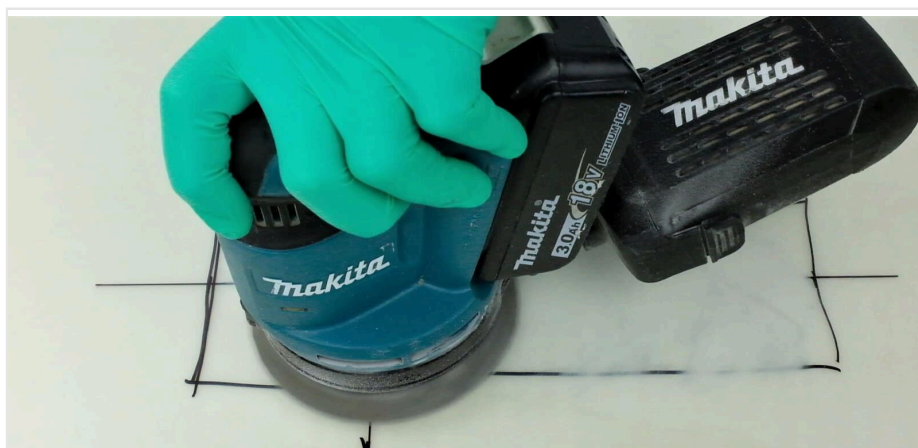
Figure 1: Grinding the installation position
