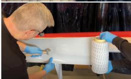
Meanwhile an operator can start from the TIP end to apply *ELLE Onshore* to the remaining part of the blade.
