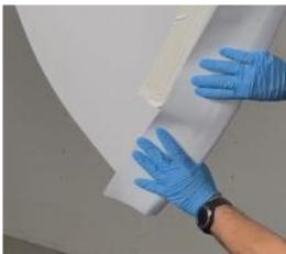
If use of the TIP template isn't necessary make a clean 90° cut at the desired length and cut a 10 mm. radius on both corners.
