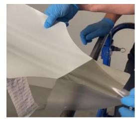
Hold the ELLE® Onshore in place without removing the liner and apply masking tape along the edges, leaving a 10 mm. gap to the ELLE® Onshore.
