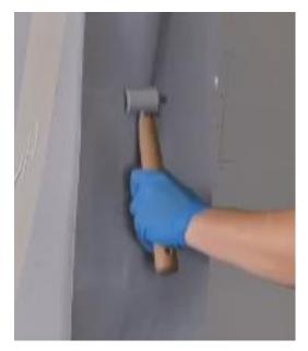
5 Stop the application and remove the loose liner material just before you reach the 0.5 meter from the TIP that hasn't been prepared.
